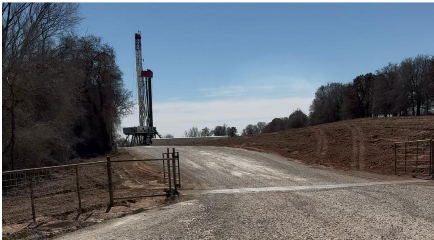
Figure 2. Bruins Well – Drilling Underway with Kenai Rig #19
