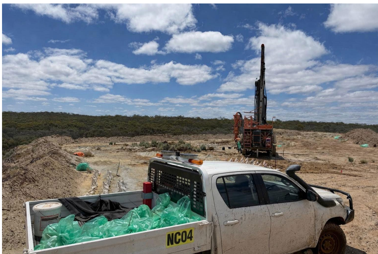
Figure 1 – Grade Control Drilling underway by VM Drilling on the Historical Stockpiles
