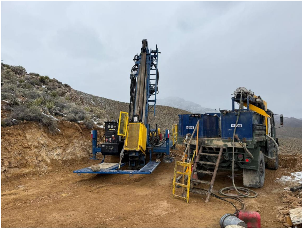
Figure 1: Drill Rig mobilised on site
