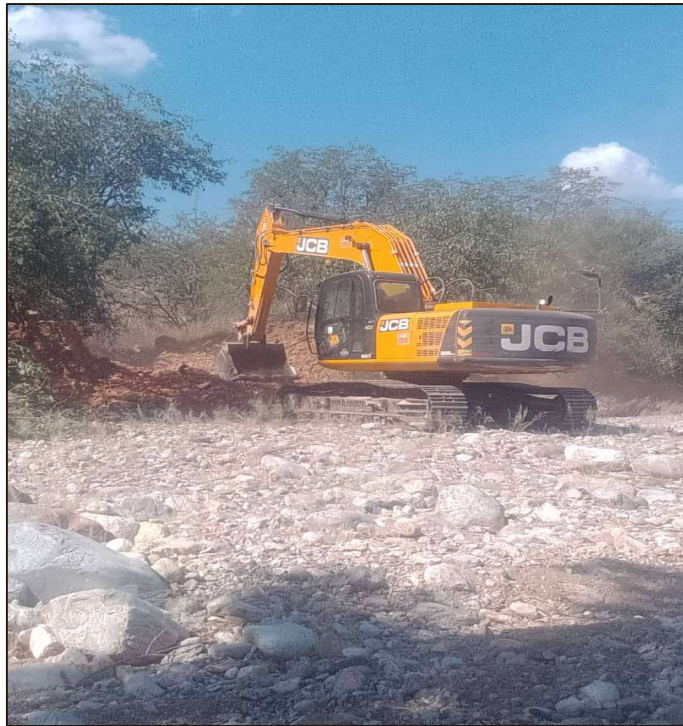
Figure 1 - Drill Readiness Works at Chalkos
