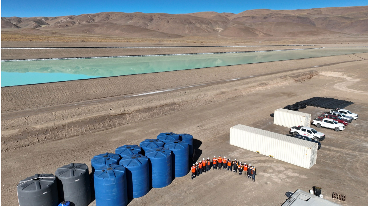
Figure 3. HMW operations team at plant site
