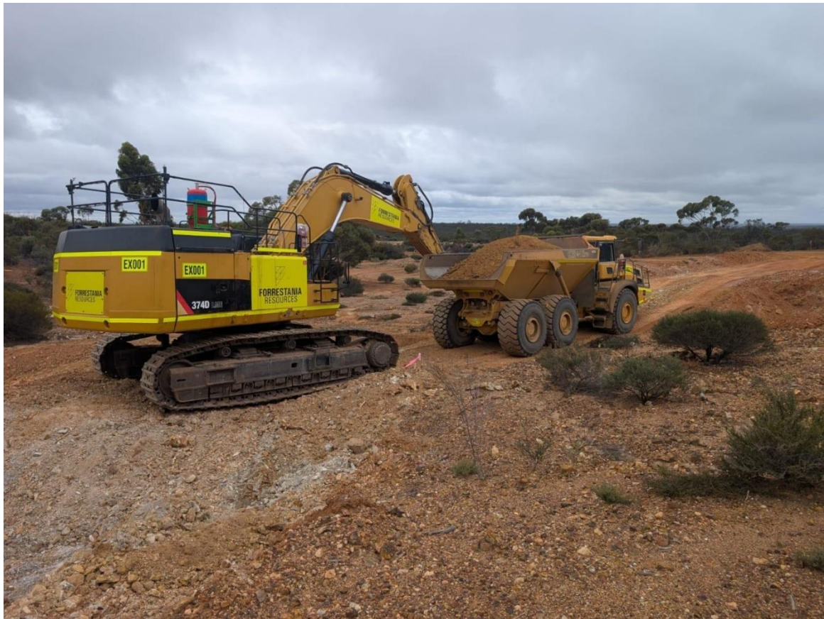
Figure 1. Ore loading with Forrester's 50t excavator
