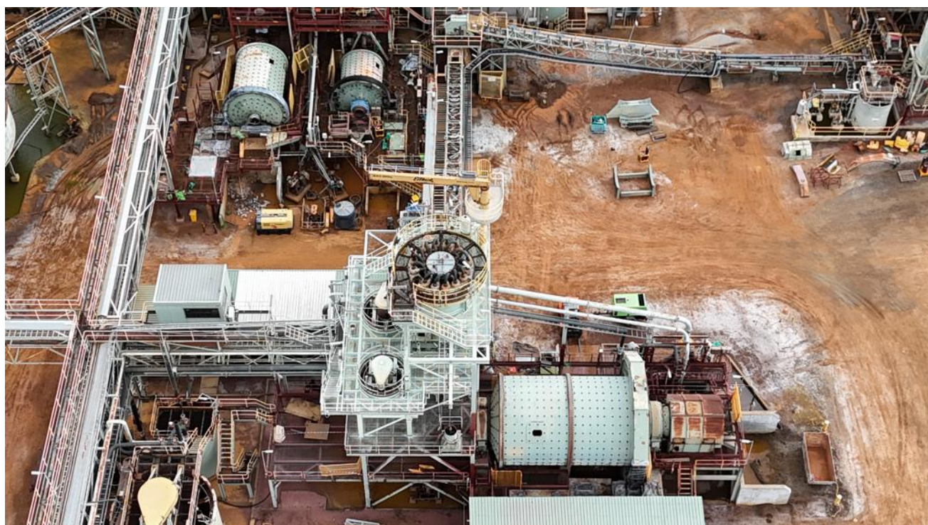
Image 1: Lake Johnston Processing Facility
