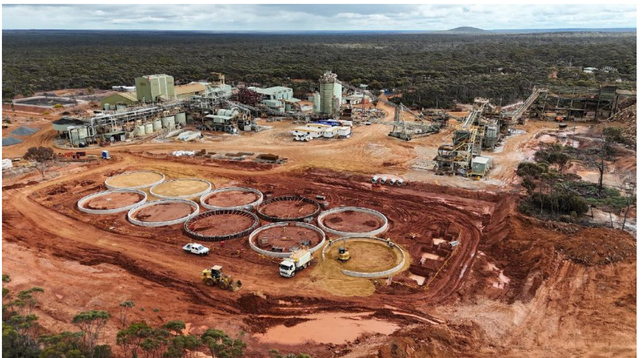
Image 3: CIL Tank construction - Lake Johnston Processing Facility
