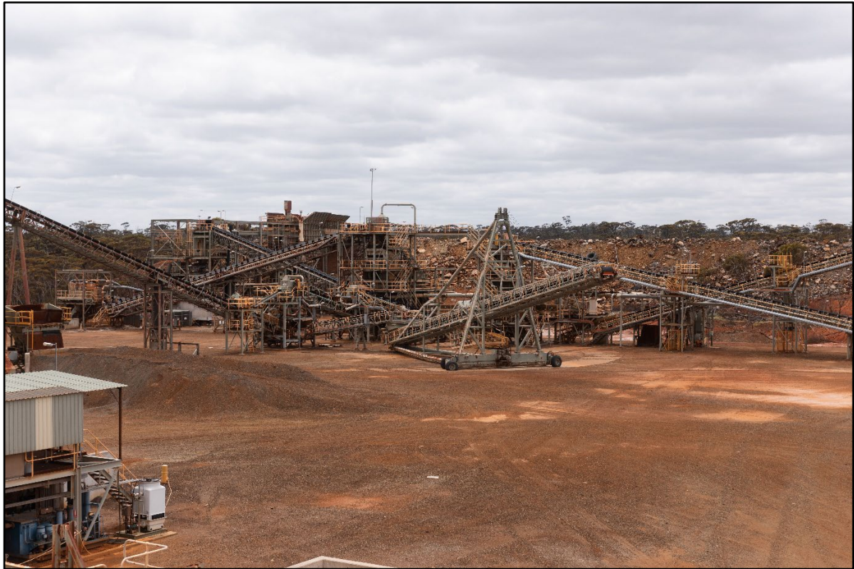
Figure 1 Existing Crushing Circuit at Lake Johnson during the ECI plant inspection.
